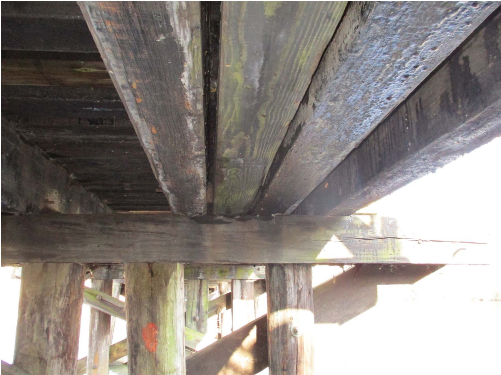
Three timber beams under past rail locations
