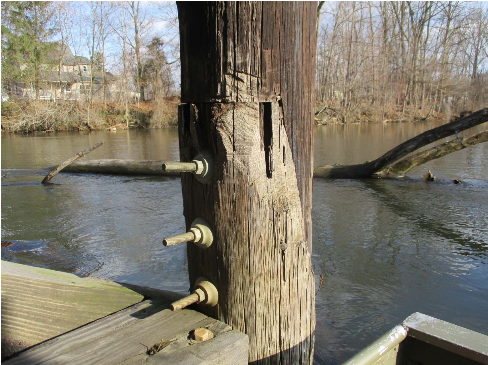
Pier 5S pile 1E bolted splice
