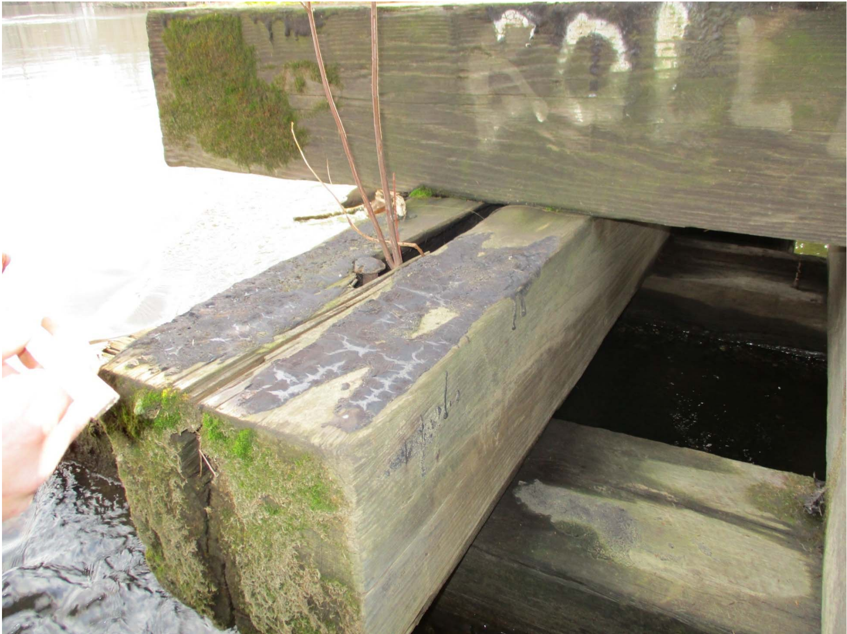
Pier 7S east end cribbing
