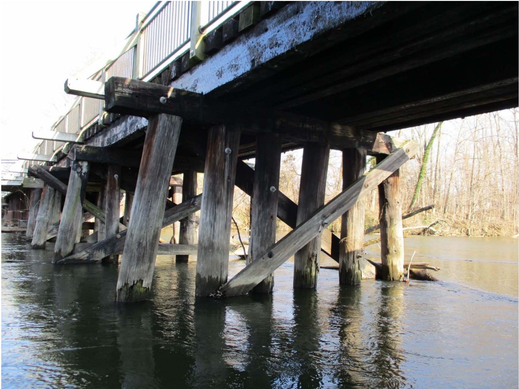
Pier 4S surface to piles at waterline
