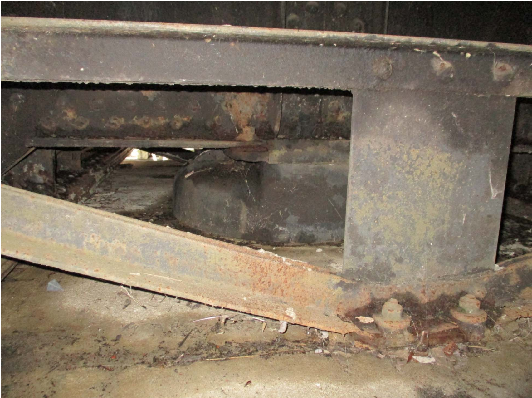
Pier 8S steel beam center support
