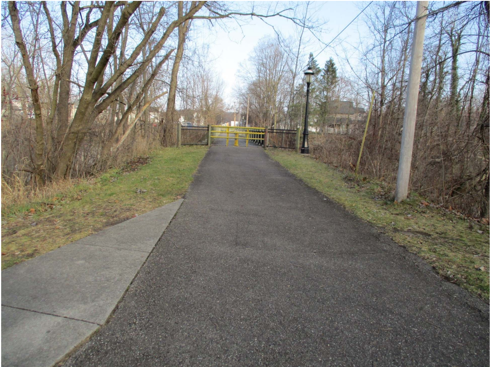
South path approach, bridge closed to pedestrians
