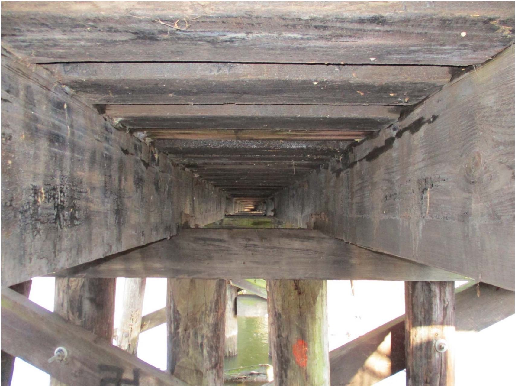
Center spacing between beams
