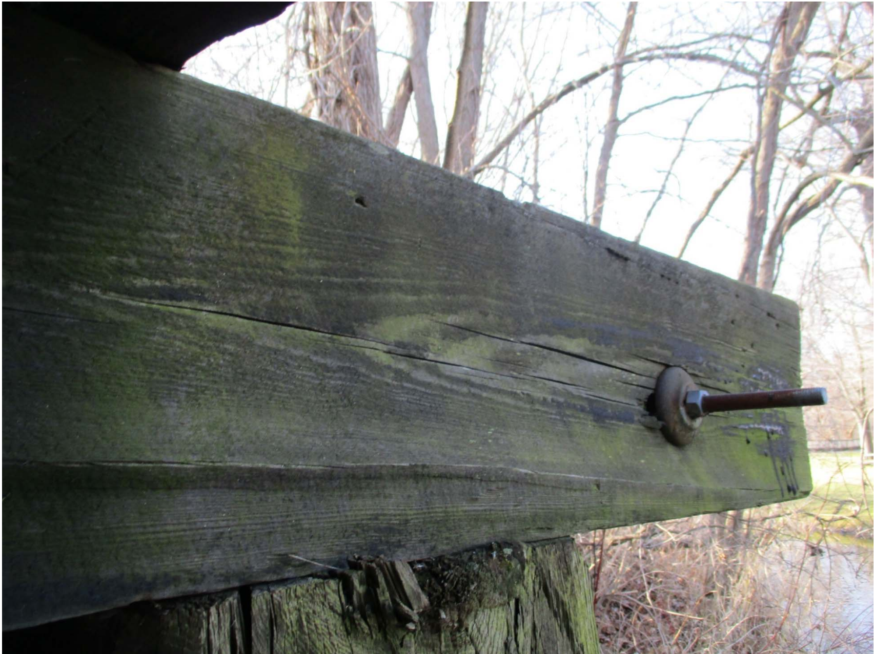
Pier 1S west end
