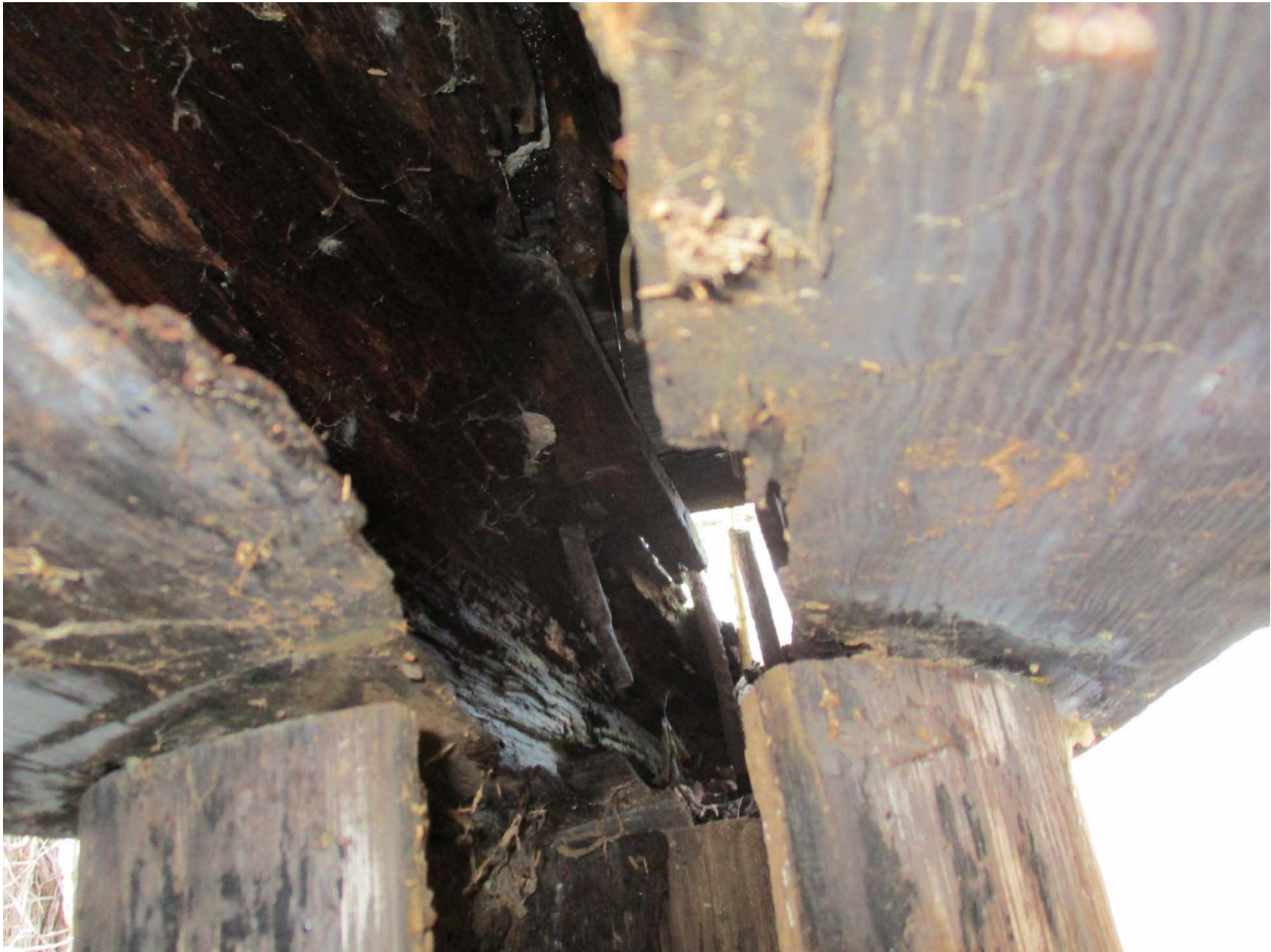
Interior view of Pile 1S west end
