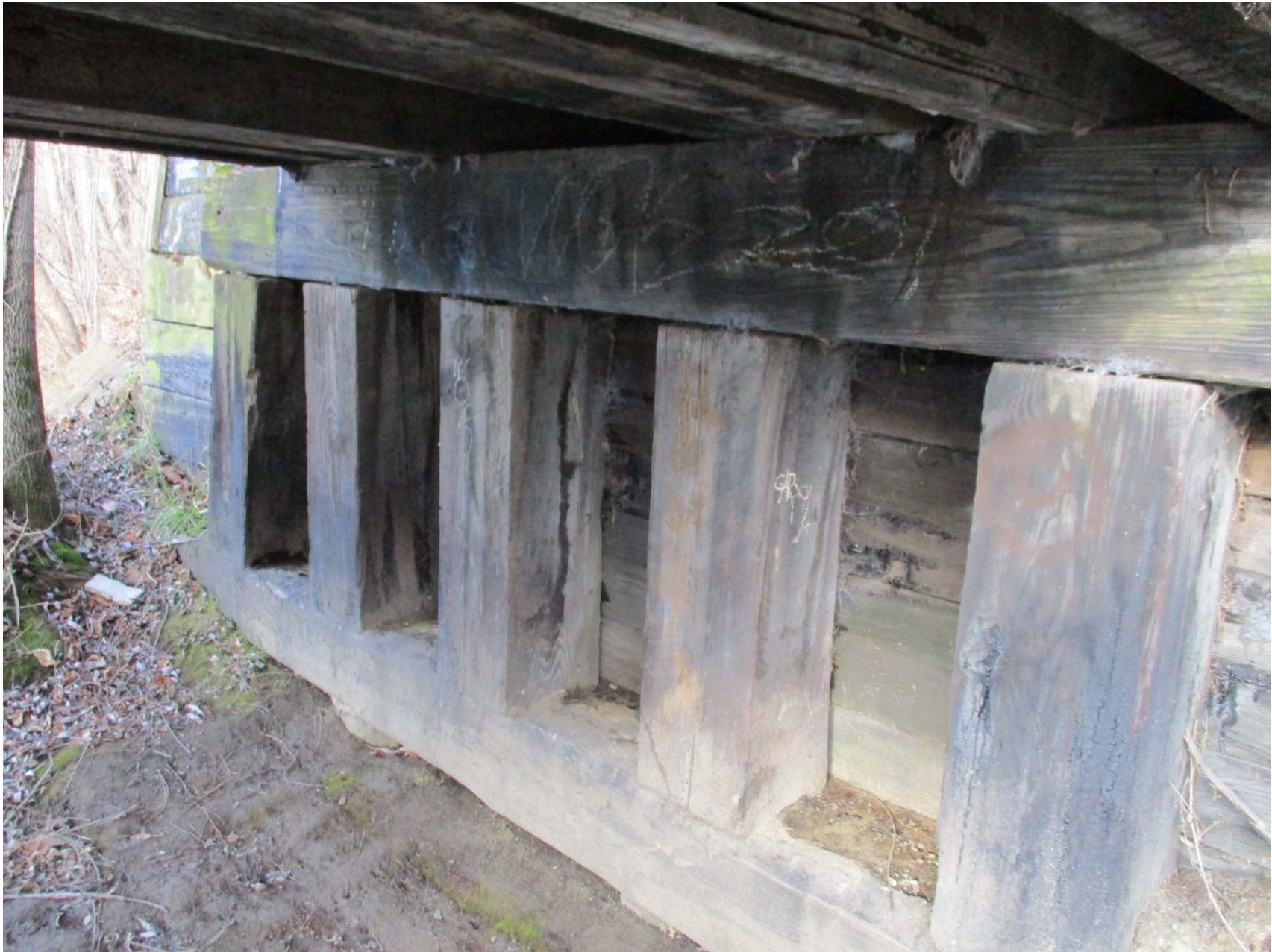
North abutment elevation
