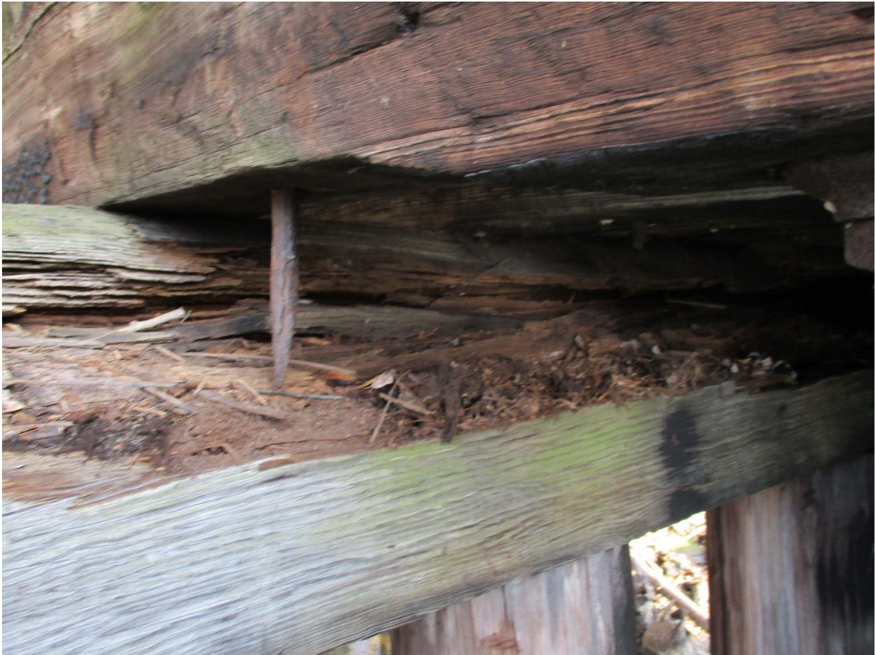
West end pier 9S cap
