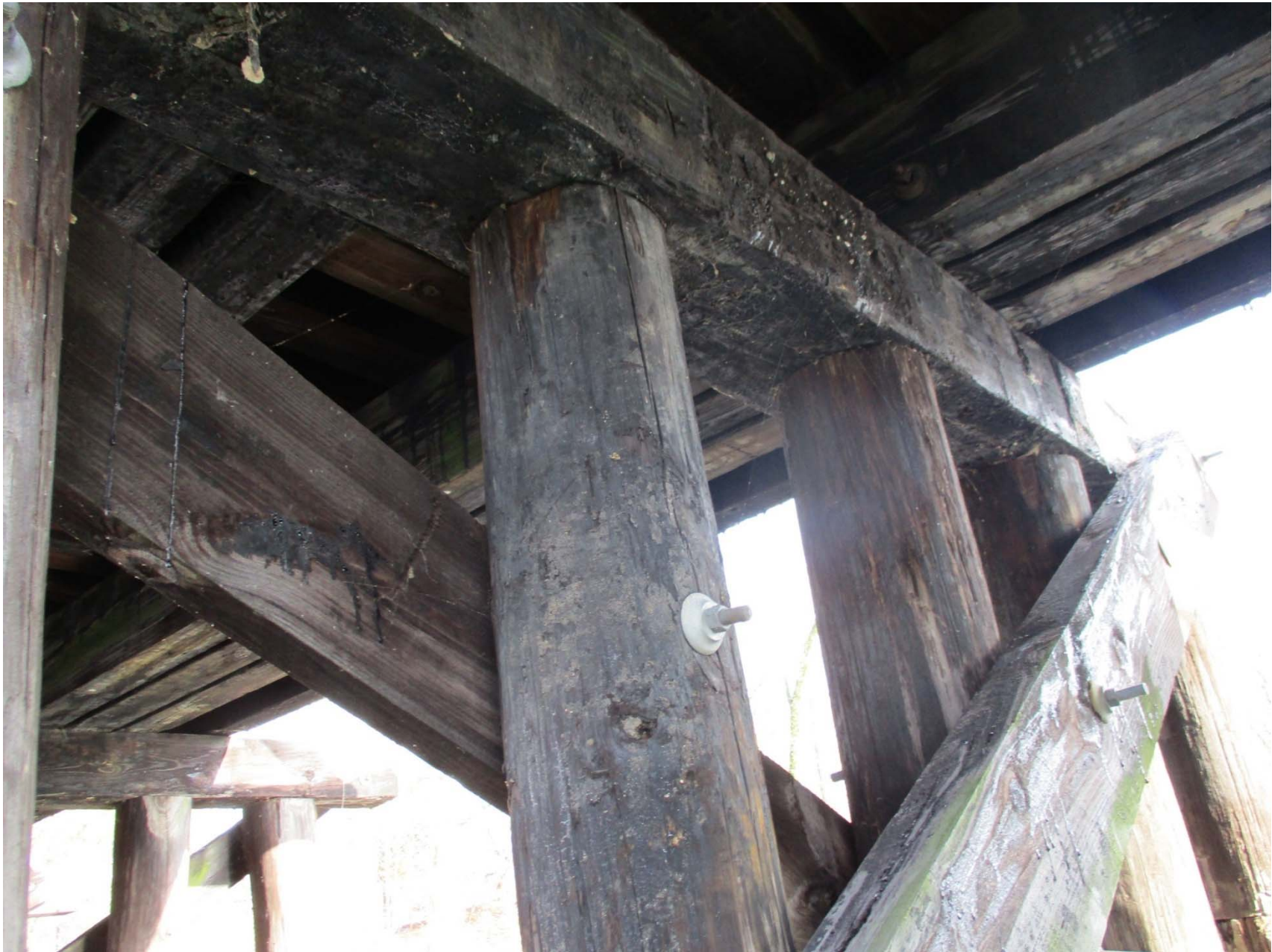
Pier 5S cap remains good
