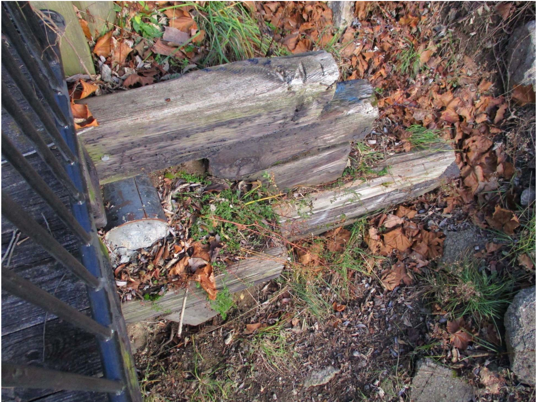
North abutment east end
