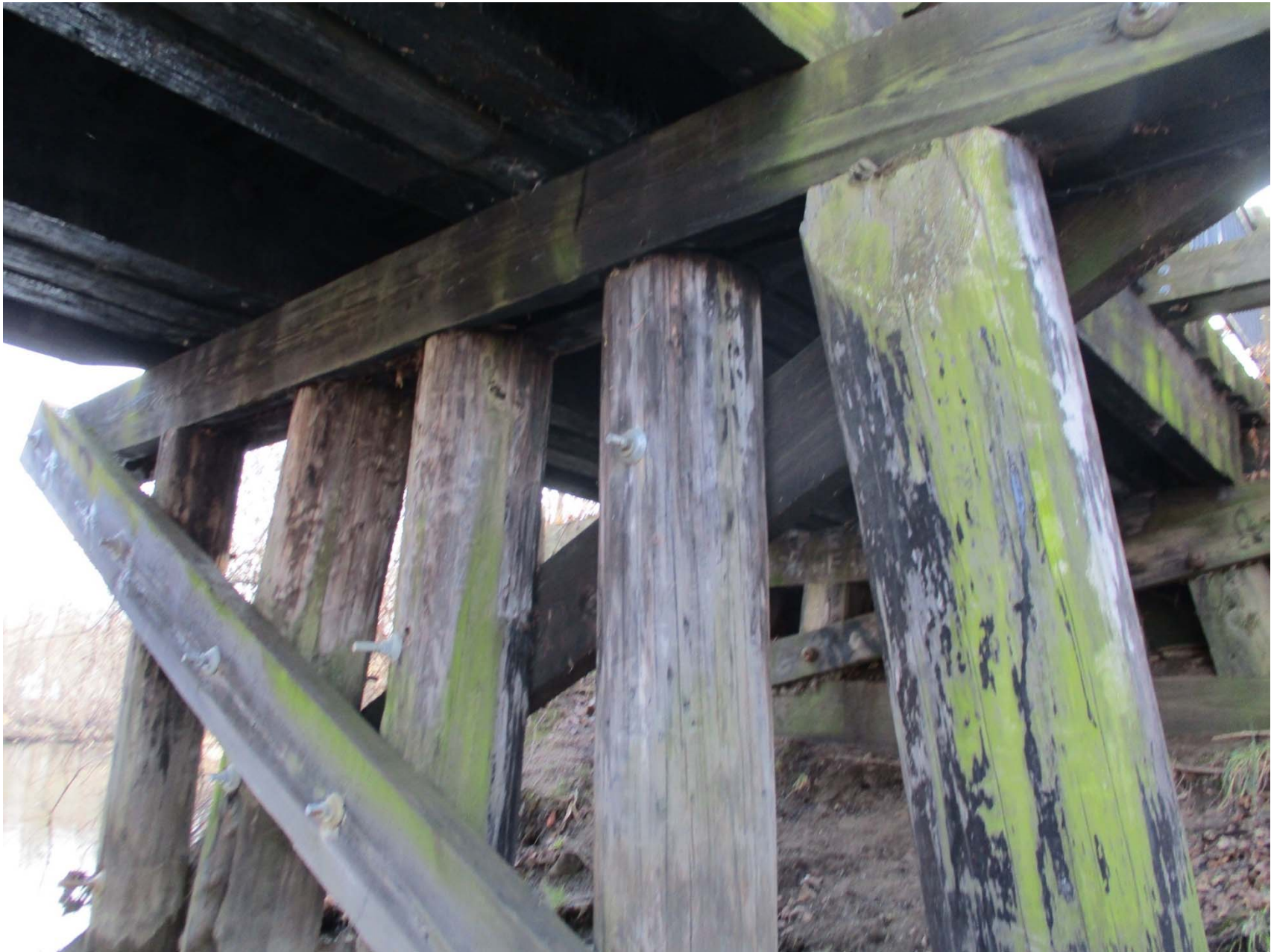
Pier 1S elevation
