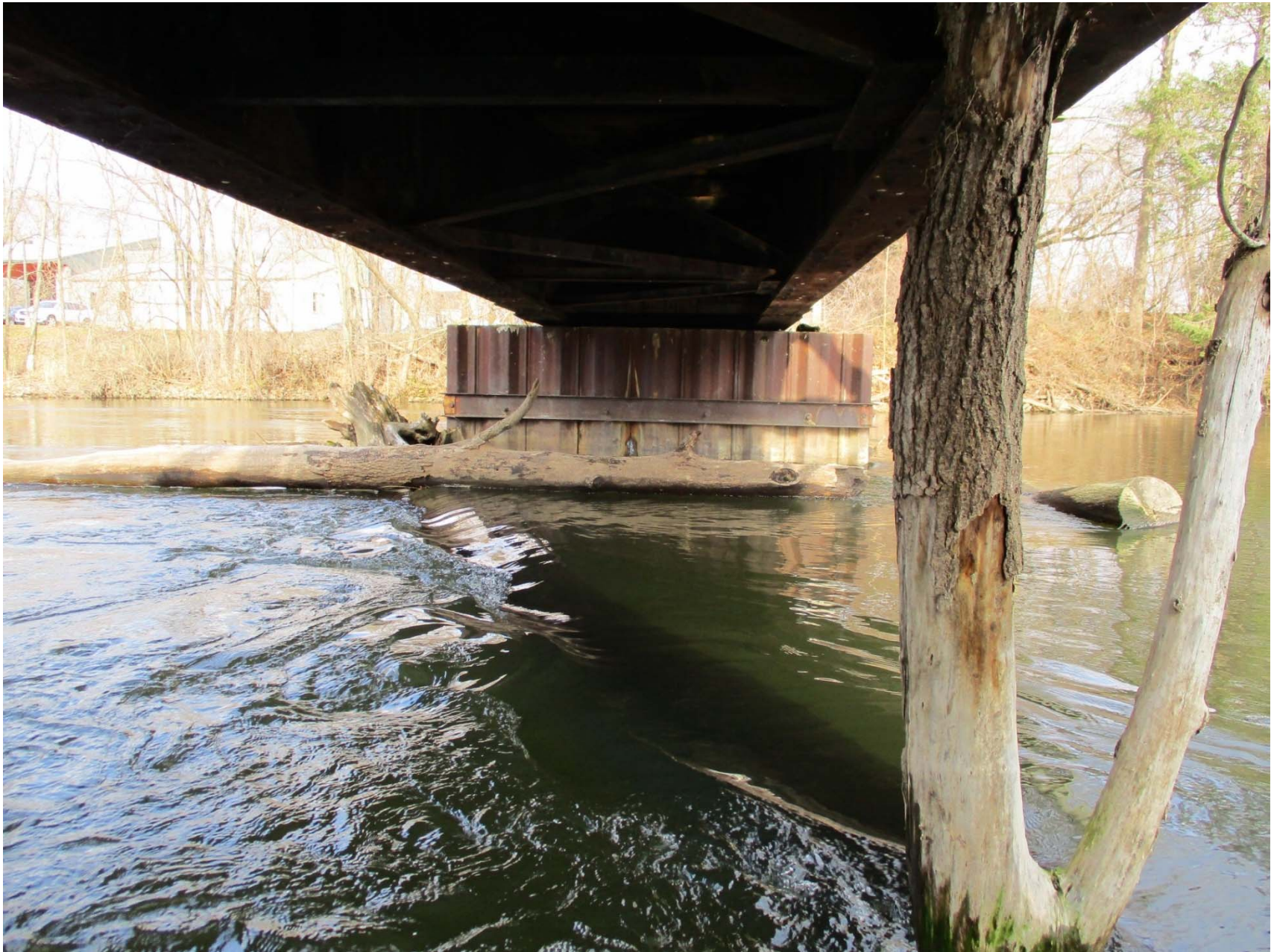
Pier 8S center support for steel beam spans
